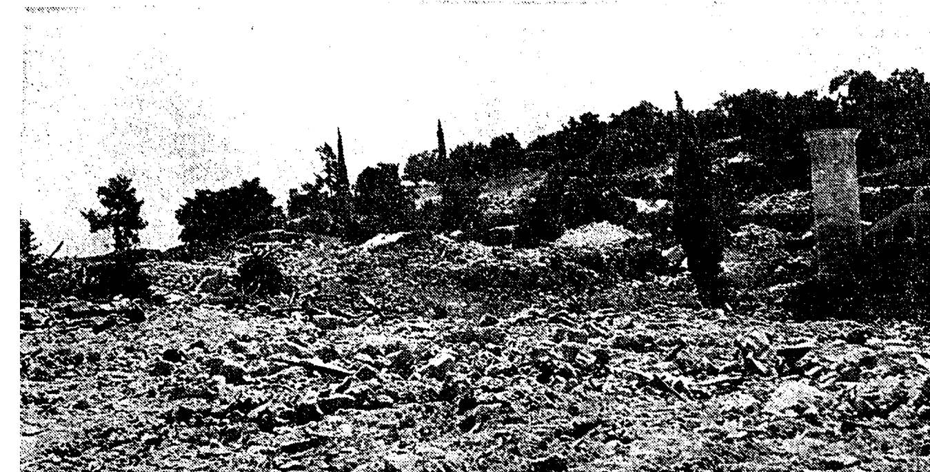
A part of the rubble of the Arab village of Imwas.
